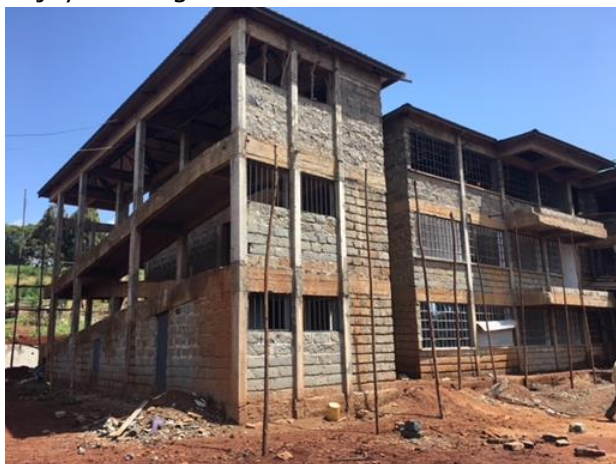
New head office of KSA in construction
