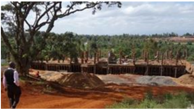
KSA main campus in Nyeri under construction
