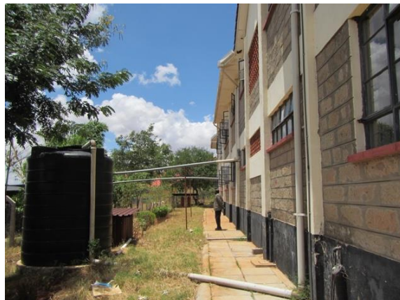
Rainwater harvesting system and collection tanks that lead to the fish ponds at SEKU campus.
