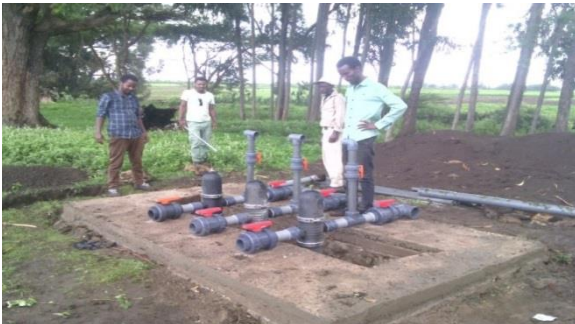
Construction of foundation base for the battery filters is completed.
