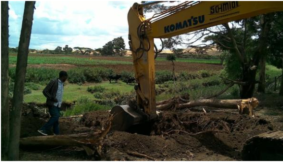
Excavation for diverting the river and sand trap construction.
