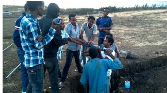
Drippers, micro tubes and watering pegs have been ordered from a foreign supplier company and are on government customs process. The installation of manifold and laterals is also completed.
