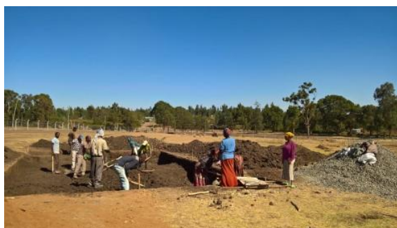
Excavation for foundation of water reservoir/ filter system (to be built).
