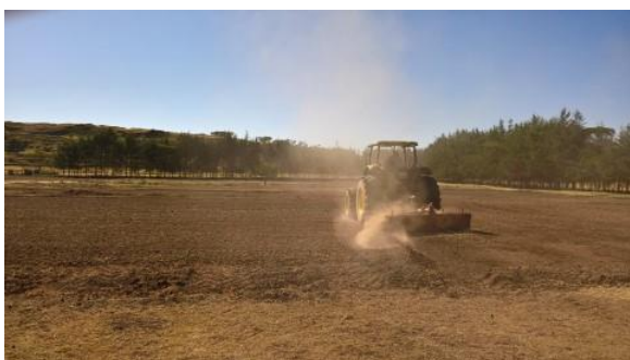
Levelling the future irrigation plot.
