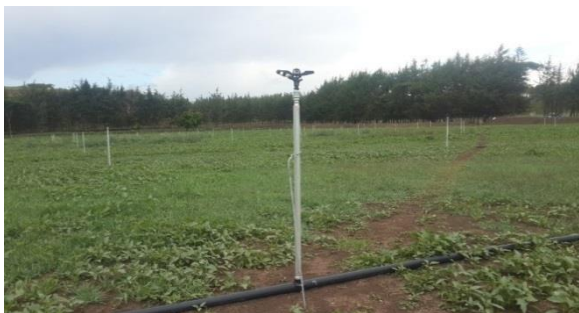
Supply and installation of all manifold and lateral pipes plus fittings is done for both drip and mini sprinkler.
